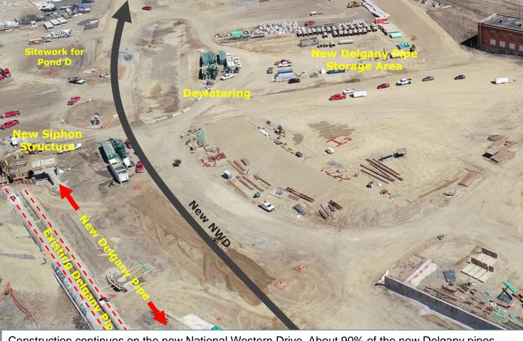
Construction continues on the new National Western Drive. About 90% of the new Delgany pipes have been installed, with the remainder being stored on-site. In this aerial view, you can see a new siphon structure, which will eventually be buried underground.
